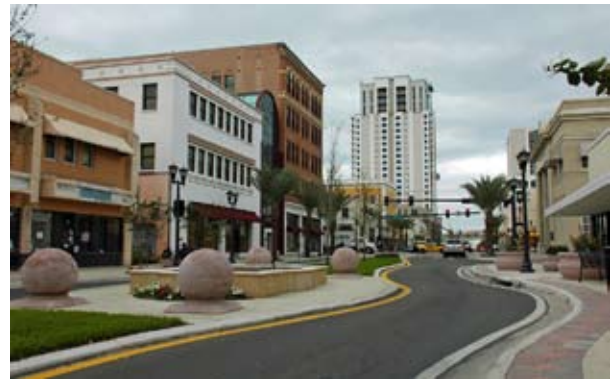
Cleveland Street Streetscape, Clearwater
